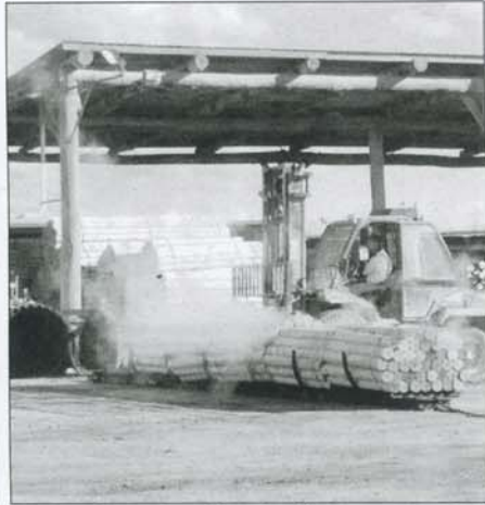
• Willmott Forests is working to install a new treatment facility on the existing drip-pad at Sandy Lane which will increase capacity of production by about 300%.
