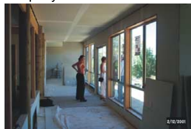
Building progress at the new Willmott Forests Regional Office & Training Centre.
